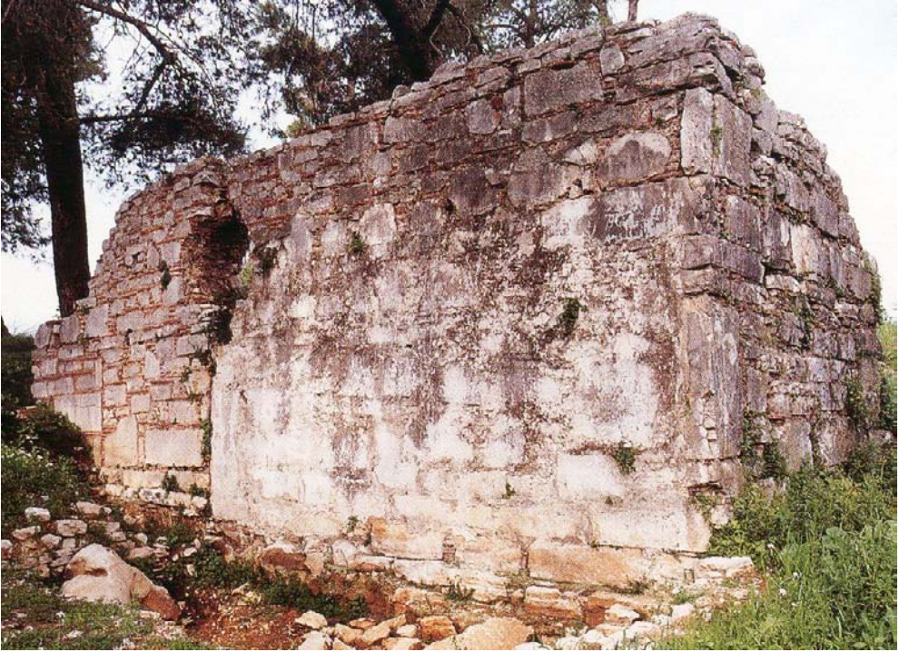
Fig. 104. Castle of Arta, SE building. View from SW.
